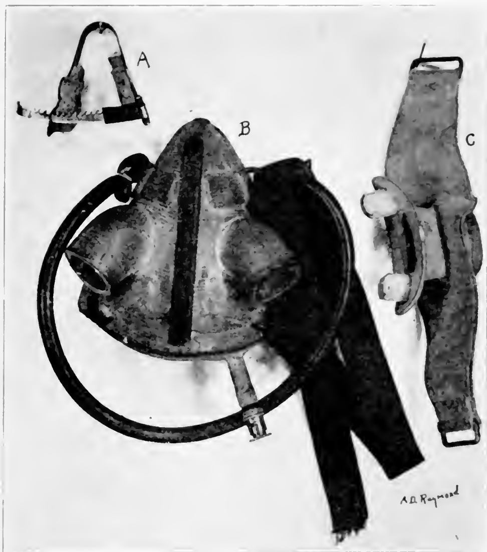
Fig. 177. A, Nose clip; B, Face mask; C, Mouth piece.
